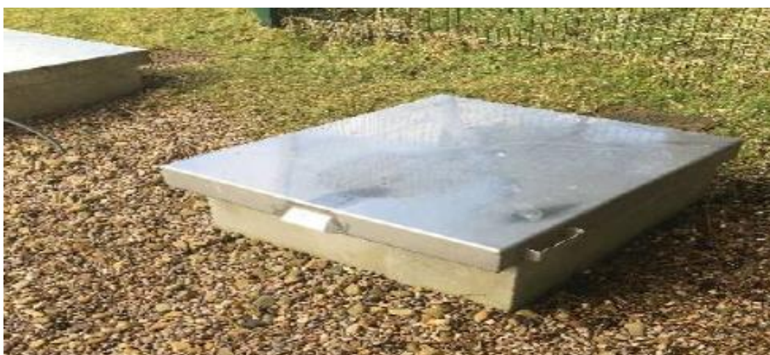
Figure 8: Hatches in good condition at Yorkshire Water's Thornseat service reservoir
