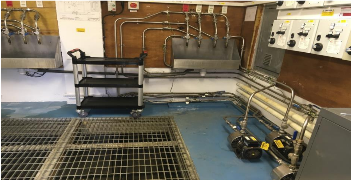
Figure 10: Clean working area by Thames Water sample point
